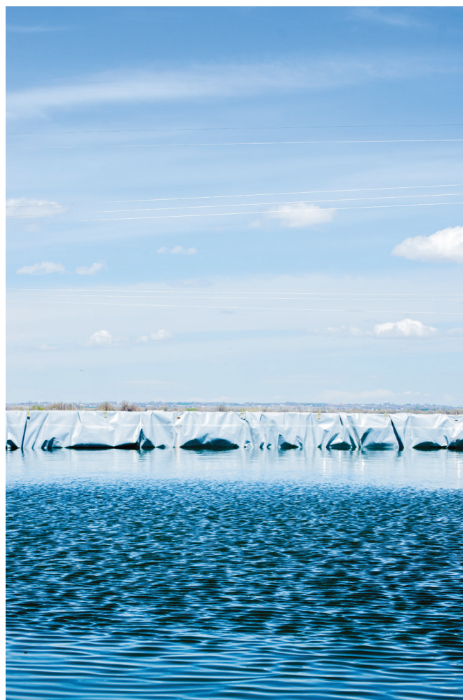
Figure 2. Pre-treated water is held in an above ground storage tank prior to hydraulic fracturing operations.
